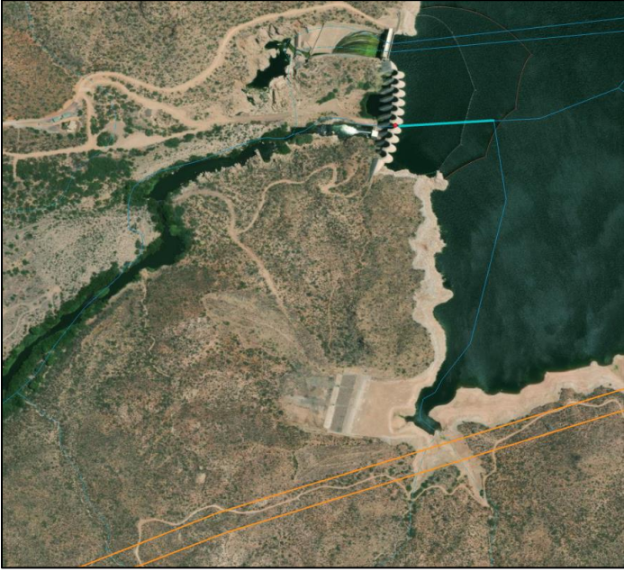
Figure 2: Zoomed in aerial view of Bartlett Dam, where we see it's buttress-type structure, and the highlighted blue line that gave us details on an annual mean flow of 692 cfs.
